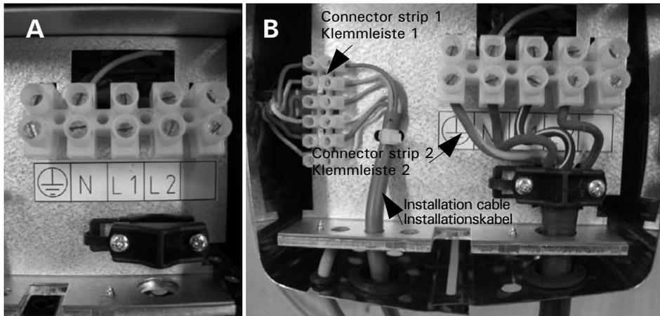
**Figure 10 A and B. 2-phase electrical connections of the heater**
