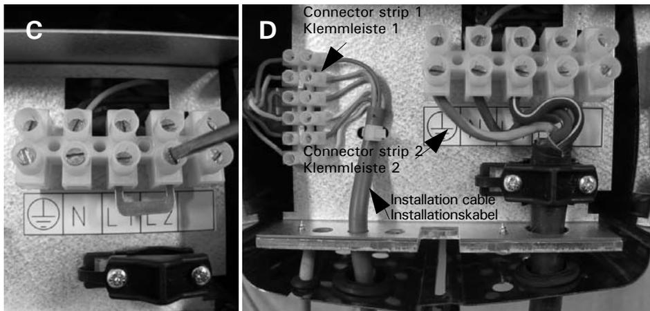
**Figure 10 C and D. 1-phase connection of the heater**
