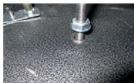
Threaded rods are screwed in ready-made thread openings in the lower part of the sauna heater. Screw the threaded rods to the depth of 50-70 mm into the bottom plate.
