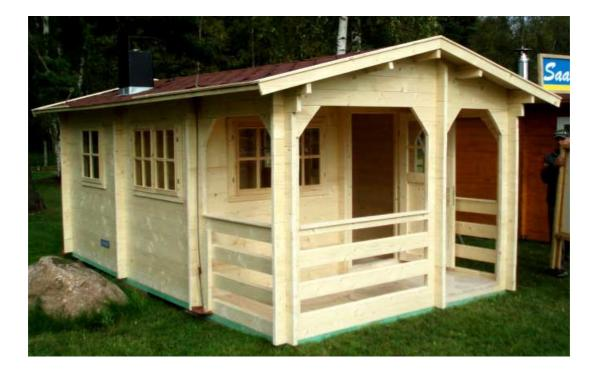
The height of the sauna house is 2,7 meters. Sauna roof covers 20,8 m2 All the sauna windows have fire protected glass TT-3 The roof also has fire protected materials of B-roof category
