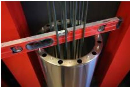
1. Straighten the sauna stove with the help of a spirit level. The spirit level can be lowered between the resistors to the lower level of the sauna stove, where you can check the straightness. Check the straightness in both directions, adjust with the adjustment feet. If no stones have been piled into the sauna stove yet, the adjustment feet can be rotated by hand, but they can also be adjusted with a 17 mm ring spanner.
