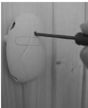
**Figure 32.** Reset button for overheating limiter
