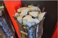
6. Pile the upper part with stones until you have reached approx. 5 - 10 cm from the top of the resistors. Lower the upper resistor plate in its place, and finish piling stones in the sauna stove. Ensure that there are enough stones on top. It is recommended to choose big stones for the top of the sauna stove, so that they cannot fall through the vertical profiles.
