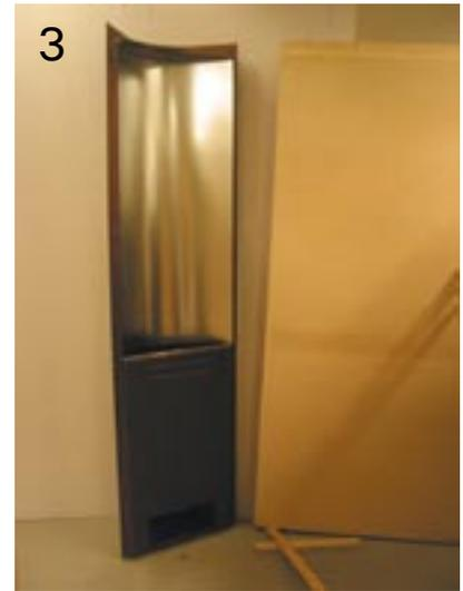
Start the installation with the back wall and back corner elements. The metal corners are equipped with "keyhole" –openings (pic 1) and the wall elements have screws which will fit into the openings (pic 2). Using the wooden sticks included in the delivery, lift the wall element so that the screws can be placed into the openings (pic 3, 4 and 5). Fasten the metal corners to the wall element by tightening the screws. (Pic 6.)
