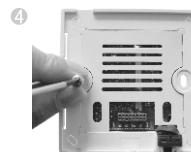
When finished,put it into back box,fix it with screws.
