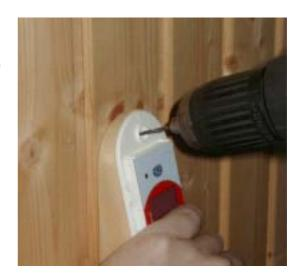
Then fix the controller using a screw to the wooden base. Once you have ensured that the controller is straight as regards the base, drill through the lower plank and screw the controller also as regards its lower part.
