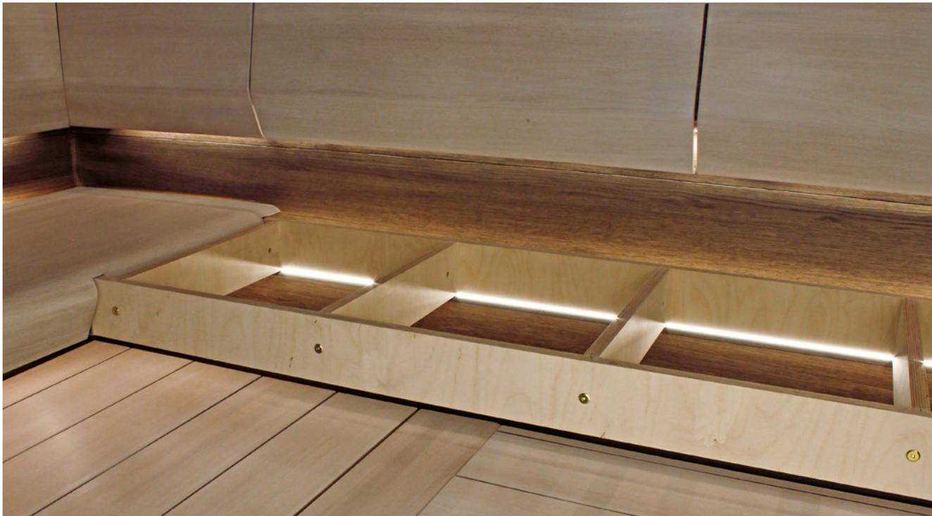
The bench units can be removed, only the frame remains. It makes the cleaning easy.
