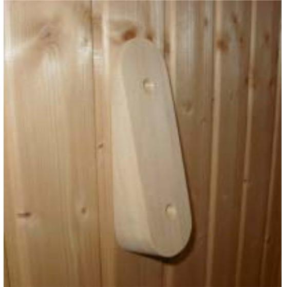
2. Place the controller as accurately as possible on the wooden base and drill a 2 - 3mm hole through the upper plank to the wooden base. The depth of the hole has no significance as its purpose is to ease the turning of the screw to the wooden base.
